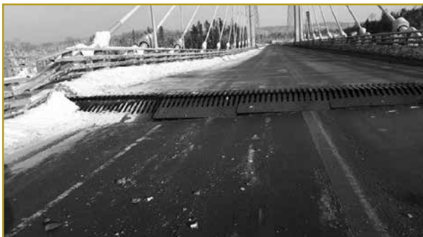
Figure 10: Nipigon River Bridge After It Malfunctioned
