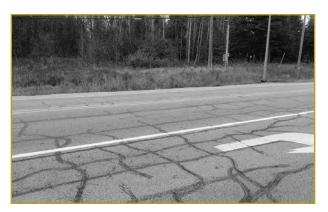
Six-year-old highway with premature cracks, in Coldwater, Ontario.
