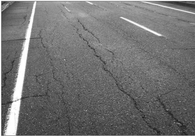
Figure 4: Asphalt Surface on a Bridge Deck Top Showing Deterioration
