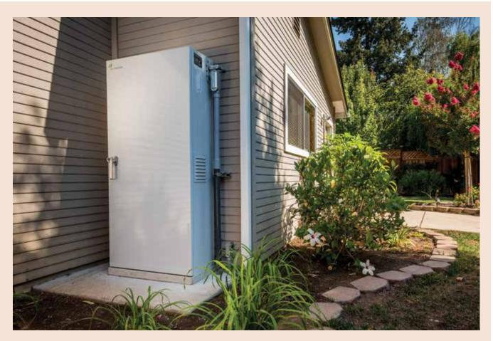
Sunverge's residential solar electricity battery storage system used by Alectra Utilities in their Power.House demonstration project. Source: Sunverge
