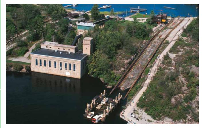
Multiple use of waterways for hydropower and navigation – Big Chute on the Trent-Severn Waterway. Source: Ontario Power Generation.
